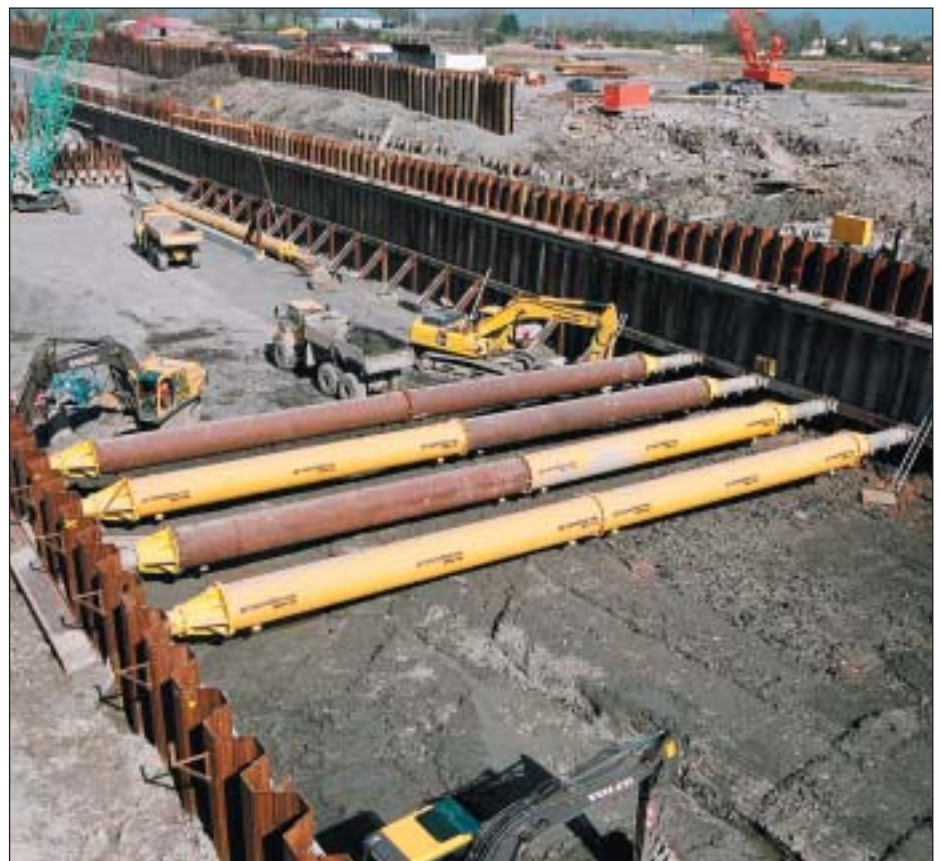
Limerick Shannon Tunnel: Groundforce MP250 struts - temporary trench support
